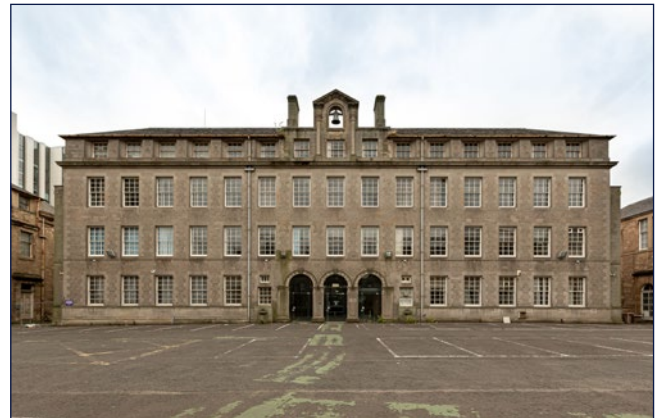
Former High School of Glasgow, Elmbank Street
