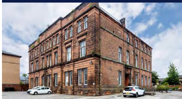
Former Napierhall Street School
